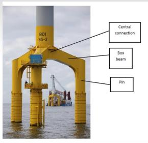
Pins, box beams and central connection are welded structures. The structure presents mostly fillet welds in T-connections and butt welds.
